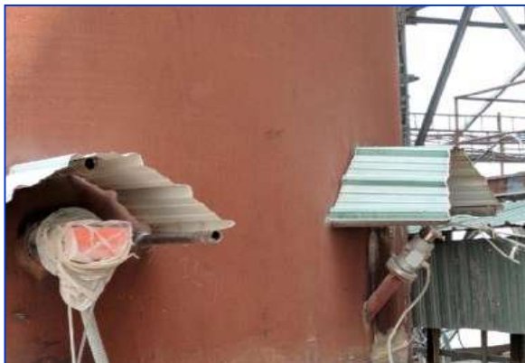
PM &amp; Gaseous CEMS for Kiln &amp; Raw Mill RABH Stack
