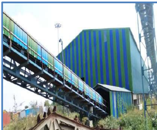
Gypsum storage shed &amp; Closed conveying system
