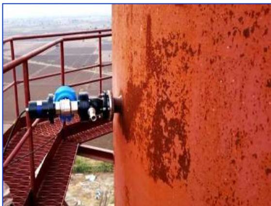
PM CEMS for Clinker Cooler ESP Stack
