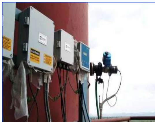
PM CEMS for Cement Mill Bag House Stack
