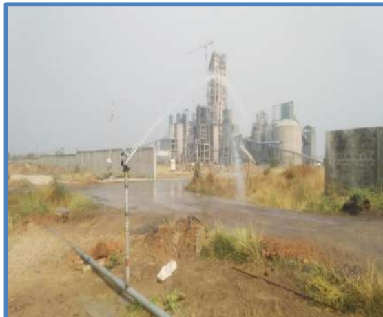
Water spraying by mechanical sprinklers
