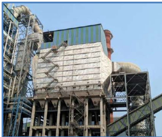
ESP for Clinker Cooler
