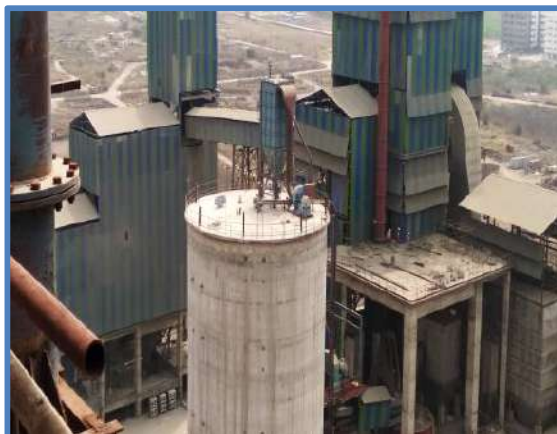
Bag Filters at Flyash silo Top
